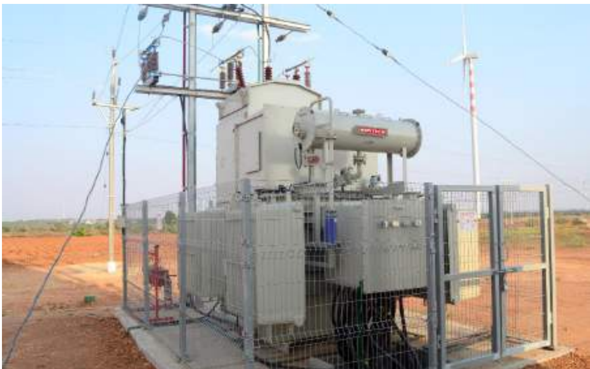
Figure 16: Skid Mounted Substation Transformer Manufactured at Indo Tech, Kancheepuram
